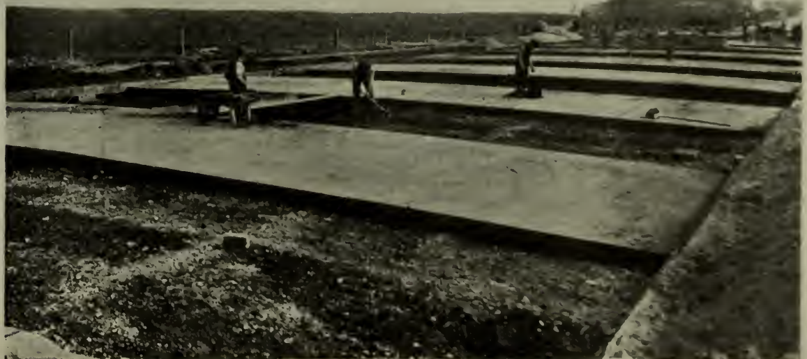
CONCRETE ROAD AT MANCHESTER IN COURSE OF CONSTRUCTION.
